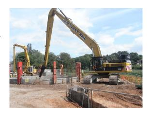
The decision was made to continue sinking the shaft as a 'wet shaft' to the full depth in order to maintain groundwater equilibrium with a base plug tremmied underwater. The standing water level in the shaft was 1m below ground level.
