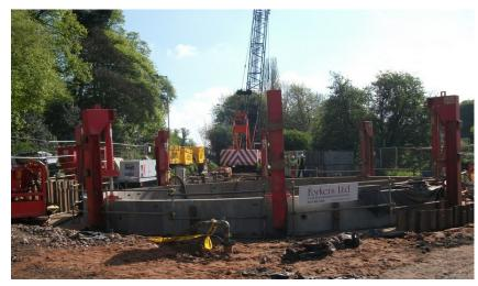
This UID project was undertaken to replace an underperforming CSO in the Compton area of Wolverhampton which, was spilling foul flow to the adjacent Smestow Brook up to 50 times annually, and was designed to intercept the existing spill pipe from the main sewer, store the first flush and then return it to the foul water system when flow conditions subside.
